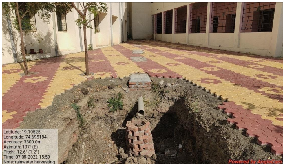
Ground Water Recharge Pit
